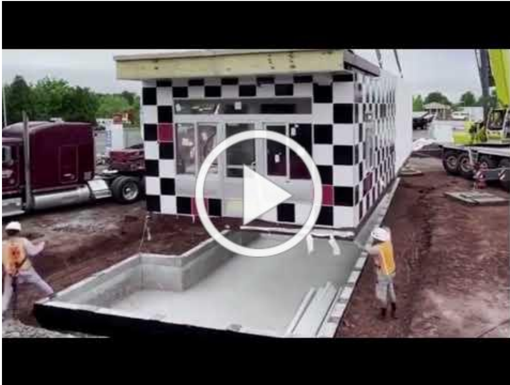
New Checkers & Rally's drive-through restaurant being dropped off by crane in Manassas on Liberia Avenue.
